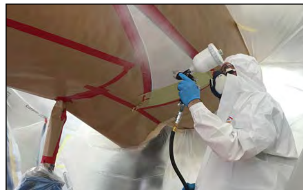
Run the filtration system during painting and curing
