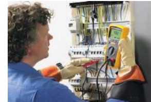
Insulation test at a distribution panel
