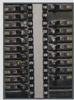
Visual inspection No issues are obvious to the naked eye.
